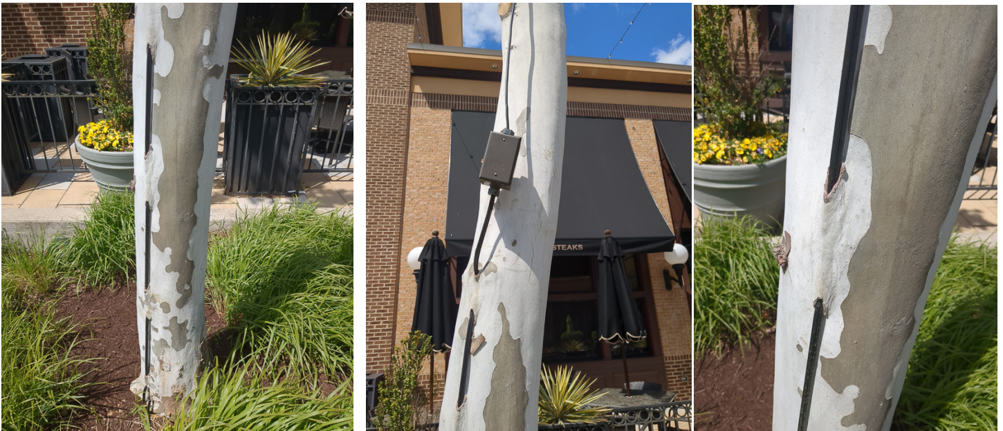
This electrical wire is completely covered in multiple places by the bark of a sycamore tree. Photos: Kyle Crouse, Howard County Recreation and Parks
